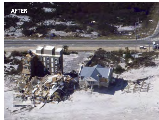
■ Storm surge can inundate structures on an eroding beach and cause them to collapse. Hurricane Ivan in 2004 destroyed these structures at Orange Beach, Ala.
