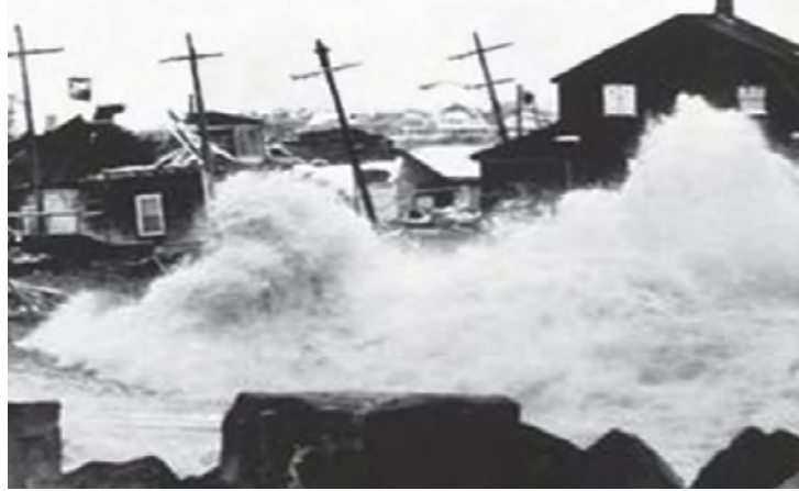
■ A storm with modest waves affecting the coast for several days – shown here in Scituate, Mass., during the Blizzard of 1978 – can cause more damage to structures and infrastructure than a much larger storm moving quickly over the coast.
